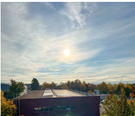
Expanded photovoltaics on the company's own hall
